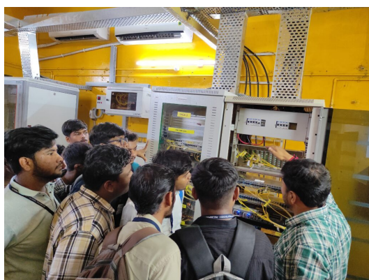
c. Railway Station, Palanpur
