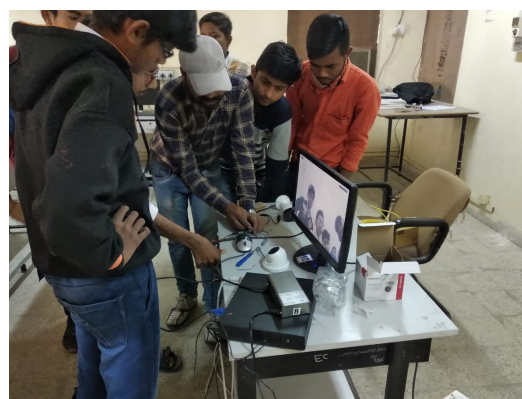
d. CCTV Installation (Contd.)
