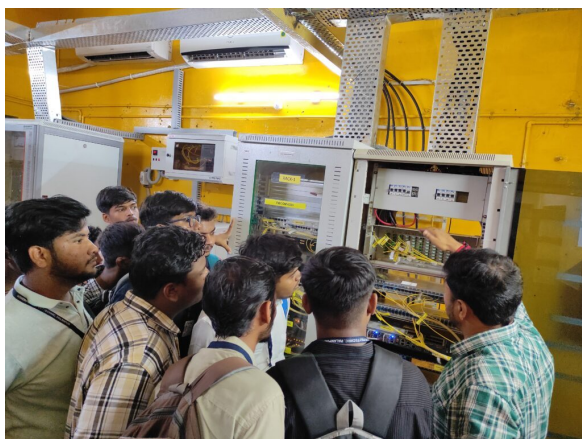
a. Railway Station, Palanpur (2024-25)
